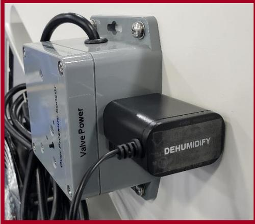
**Step 6.A Plug in Signal Cable into Overpressure Sensor**
